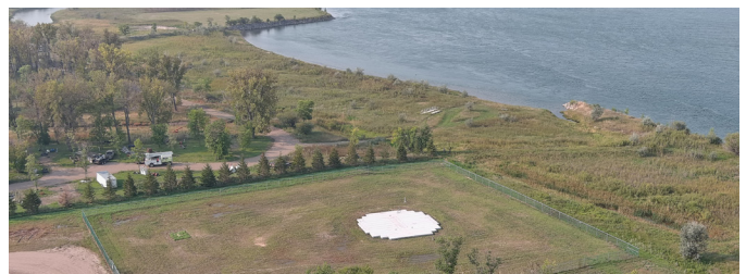
Completed Missouri River Intake
