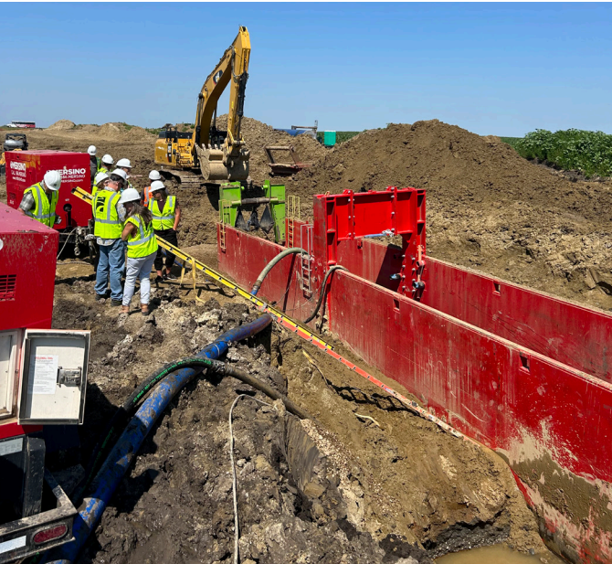
Red River Valley Water Supply Project 72-inch pipeline installation near Carrington, ND.
