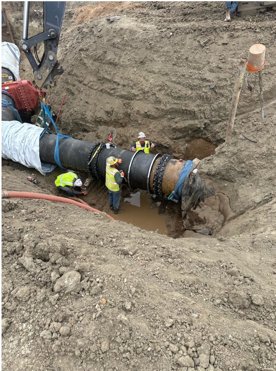
Photo 2: Contract 2-1E – Installation of Discharge Pipeline
