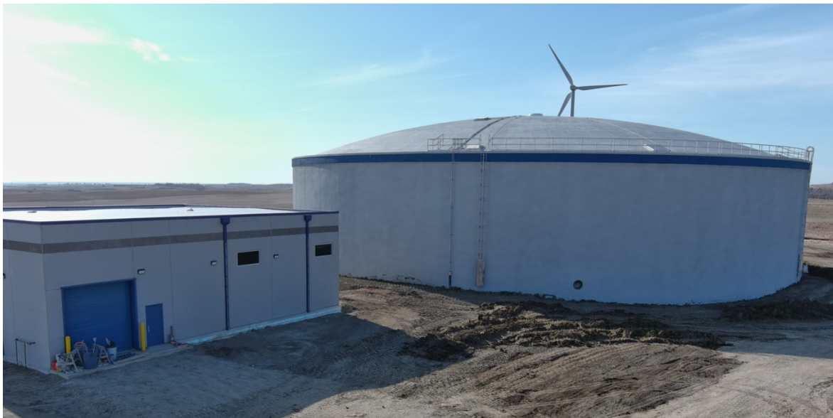
Photo 4: South Prairie Reservoir and Flow Control Structure on April 25, 2024
