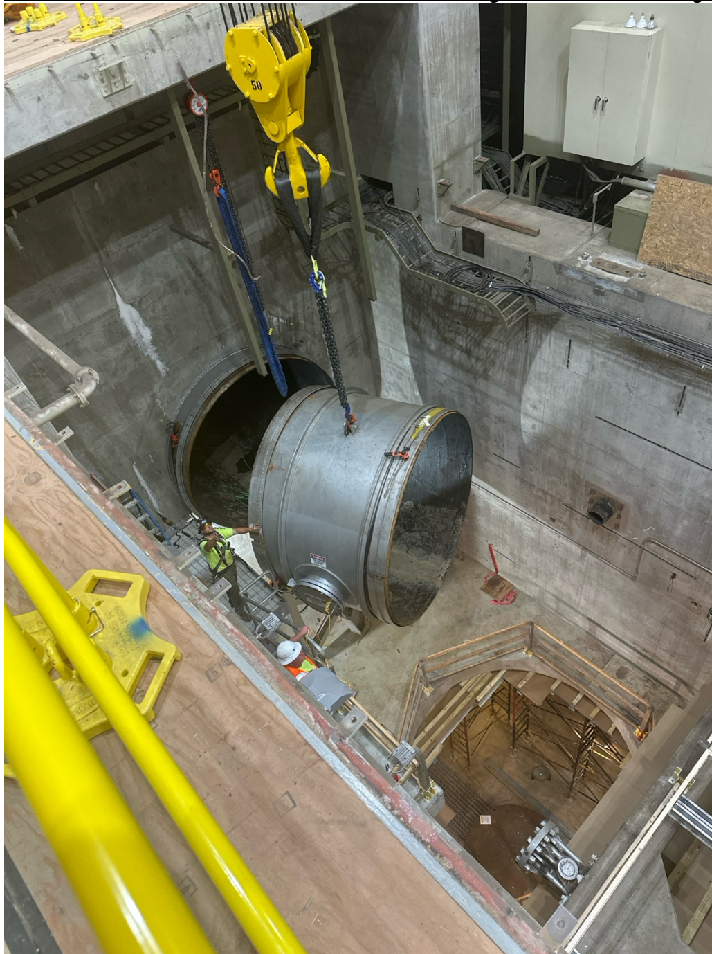
Photo 1: NAWS Contract 6-1A Demolition Contract Progress – Unit #1 Discharge Removal
