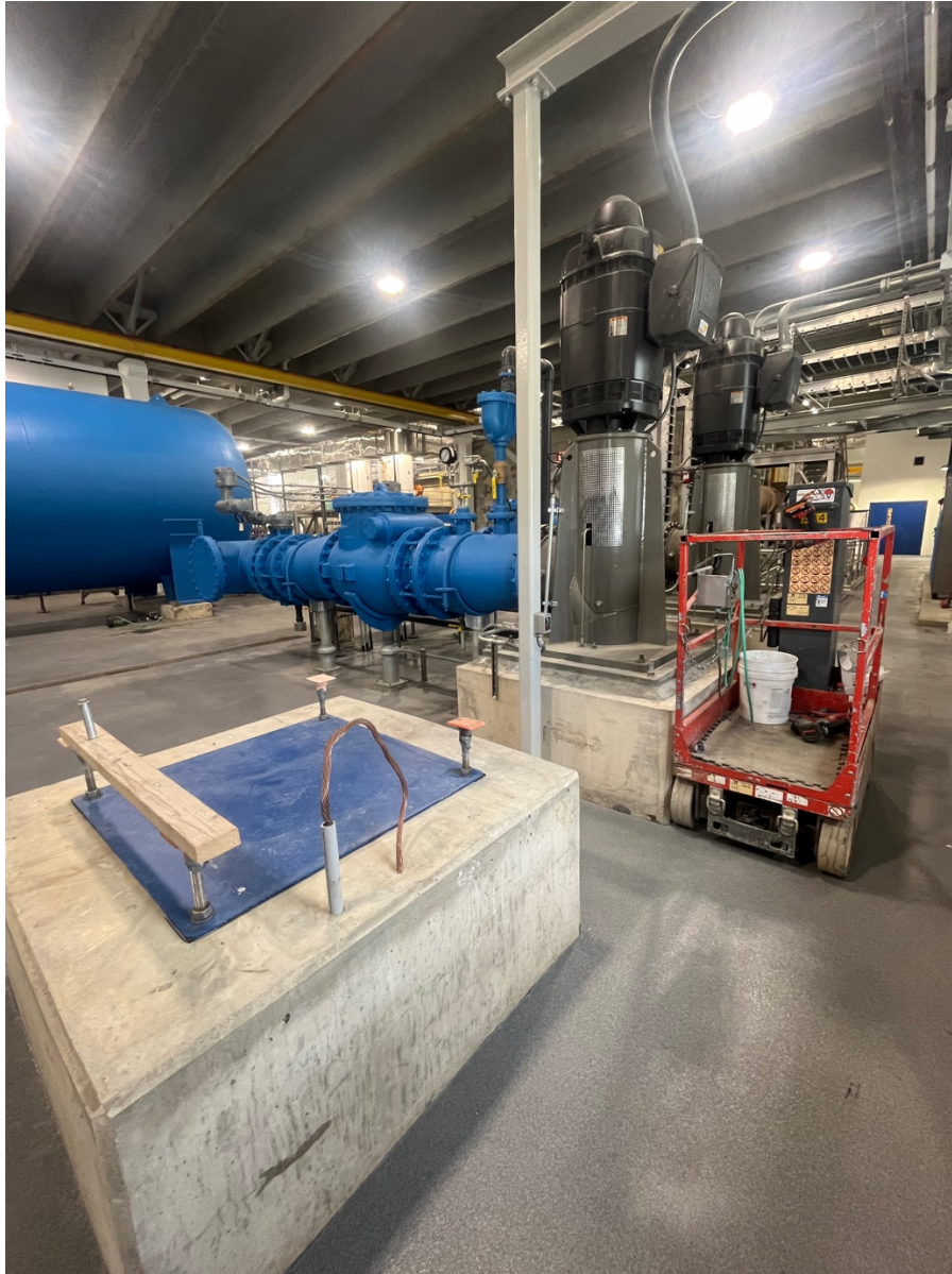
Photo 3: Biota Water Treatment Plant
