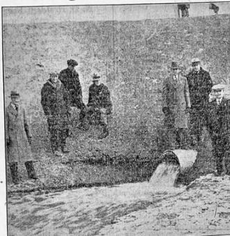
Here's water from the Sheyenne pouring into the gravel pit at Valley City which acts as the reservoir and filter for the municipal water system.
