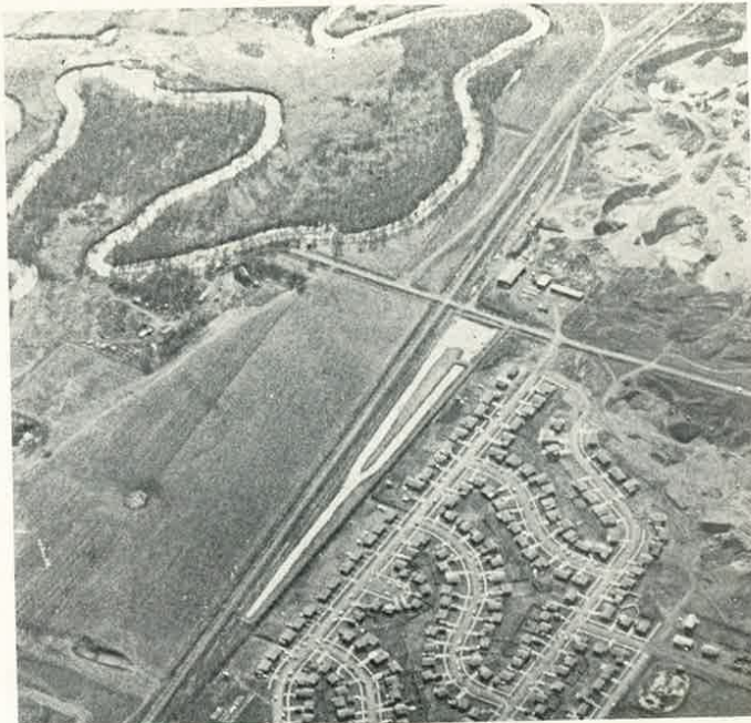
■ AERIAL view of the recharge facility, showing how it is arranged on a narrow, wedge-shaped piece of land bounded by railroad and housing near the Souris River.
